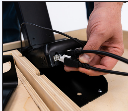
2. Connect Leg Motor Cable
